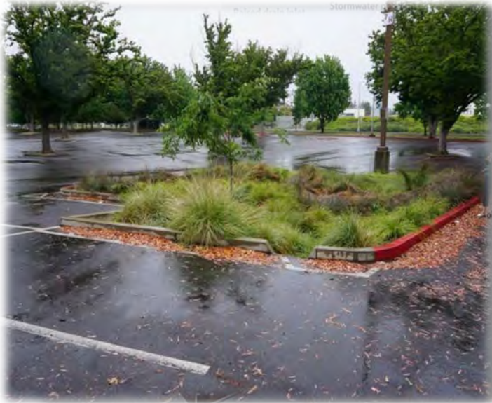
Figure A: CA State University-Sacramento Bioretention BMP
