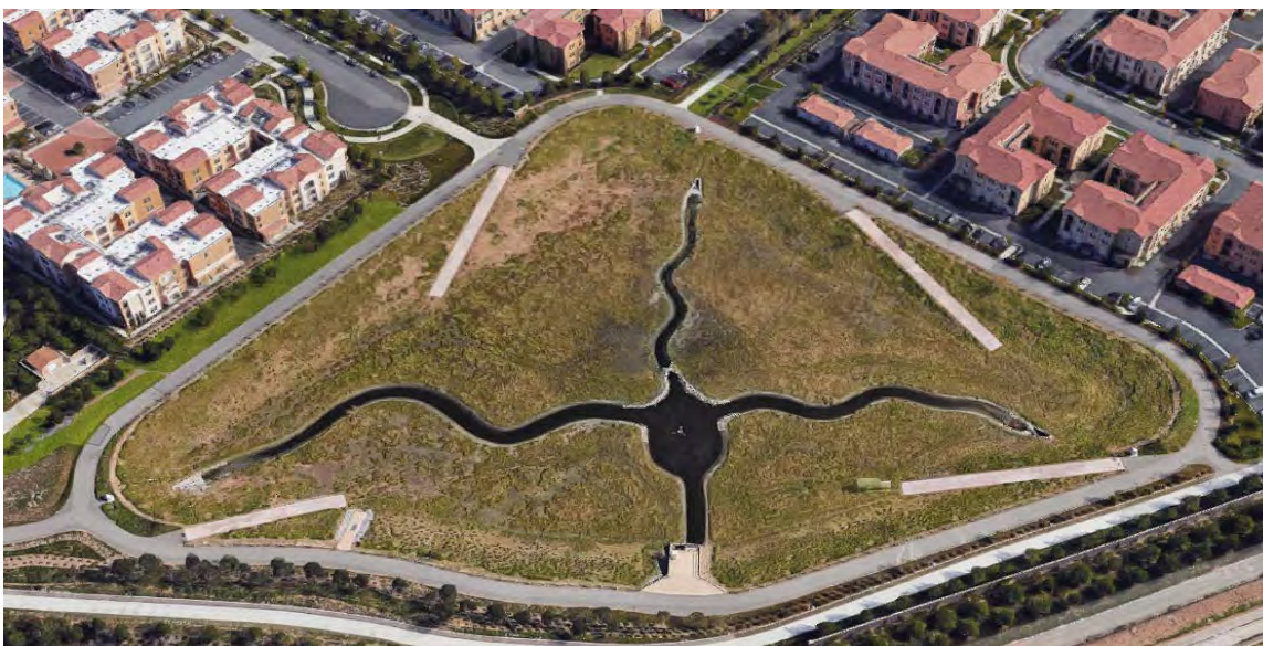
Figure A: Detention Basin BMP
