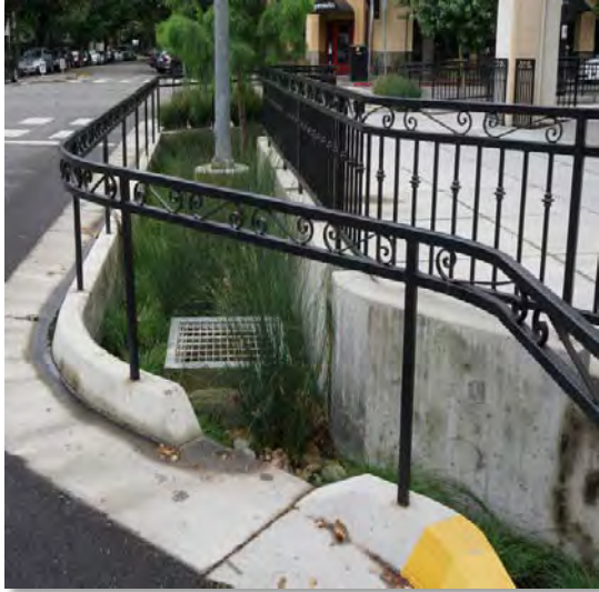
Figure A: Urban Infiltration Trench BMP
