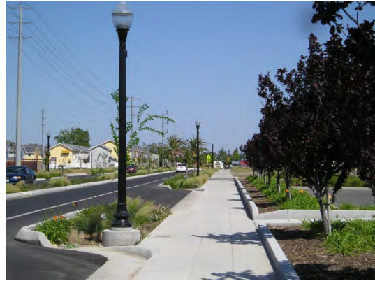
Bioretention within curb extension area - Freedom Park, County of Sacramento
