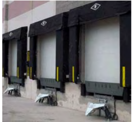
Delivery loading/unloading area. Photo source unknown
